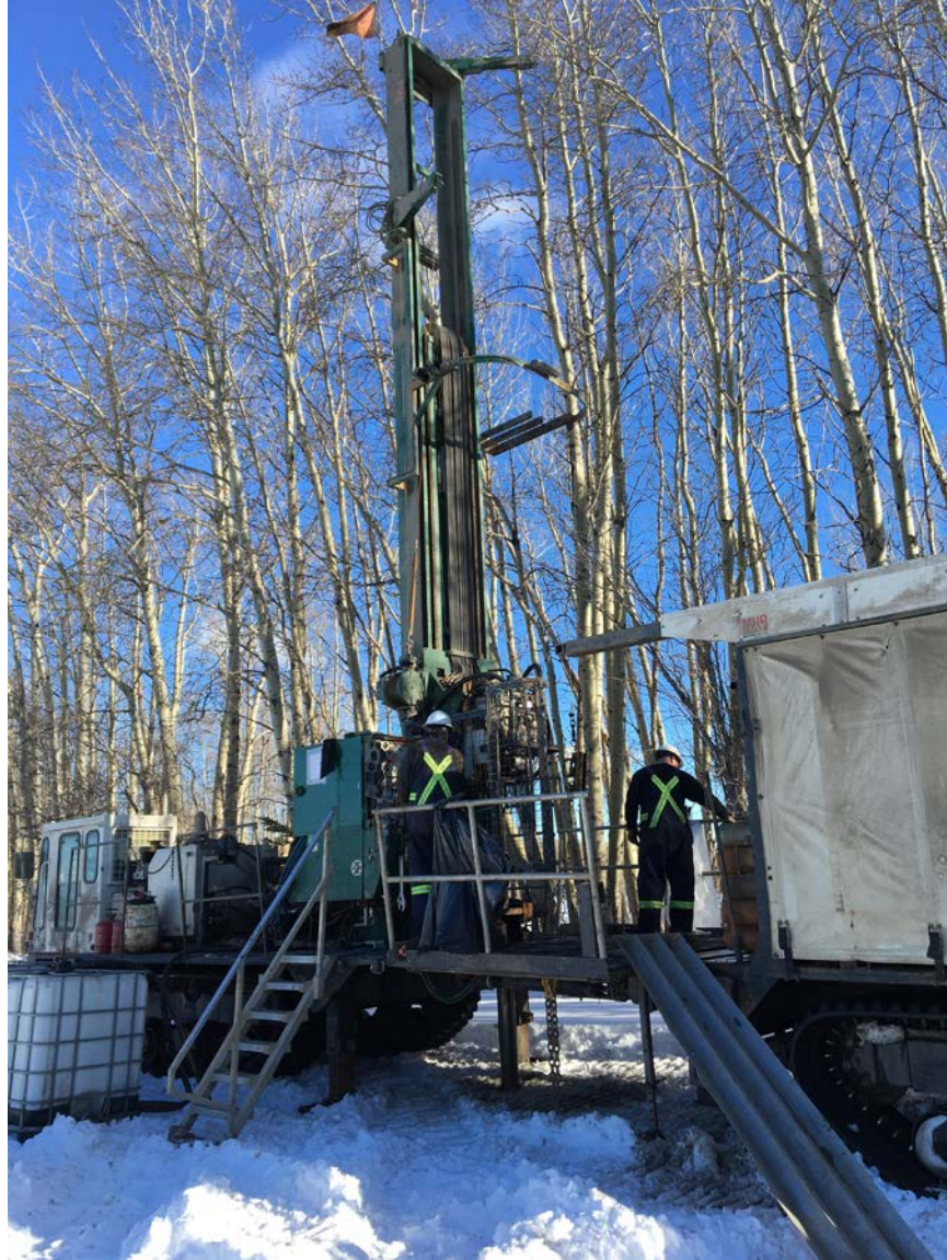
Figure 10. Sonic drill rig used during the Peace Project drilling program.
